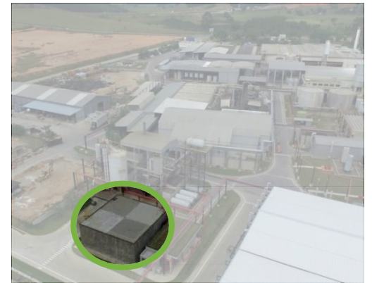
Fire Fighting Facilities (1.350.000L)
